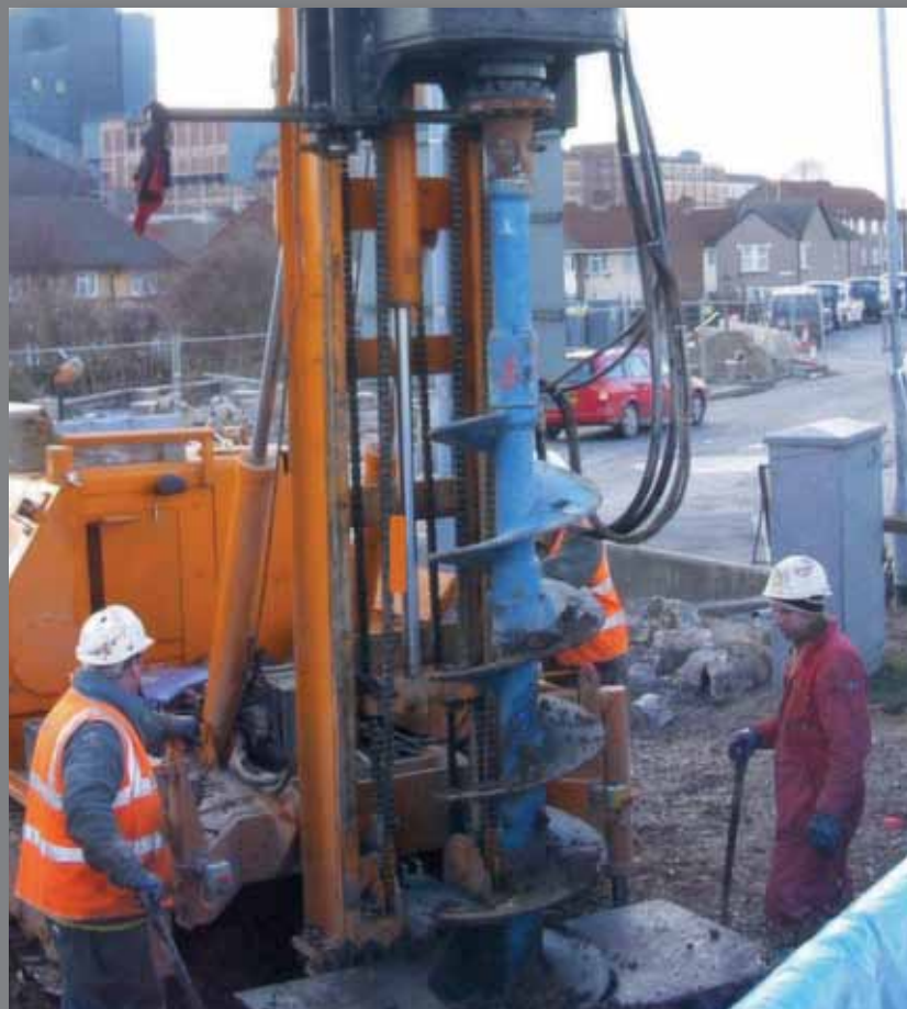
Perfuração com hélices segmentadas - Drilling with segmented flight augers
