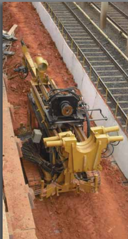
Perfuração com hollow auger - Drilling with hollow auger
